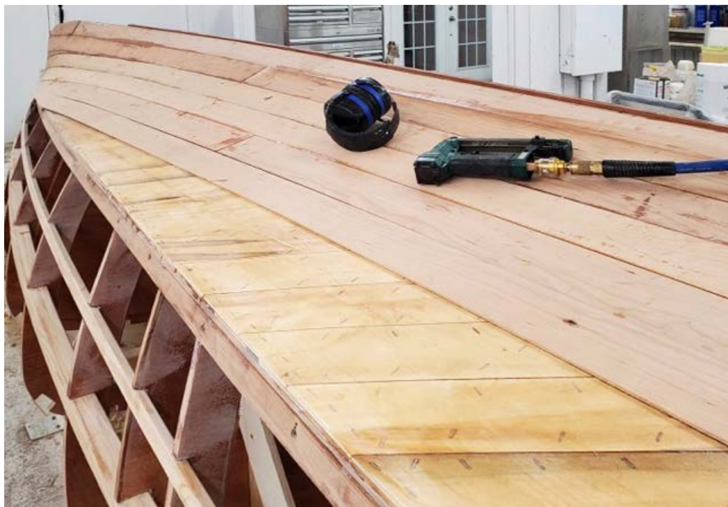
4th lamination laid fore and aft
